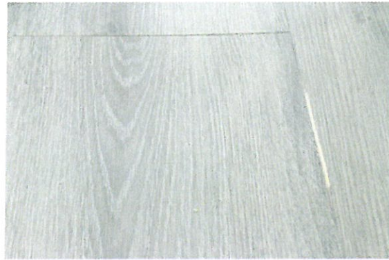
In an SPC floor, movement from above can cause the weakest point – the click system – to break as it is placed under additional pressure as in the image above.
